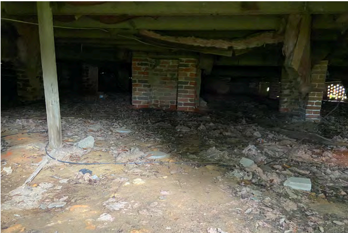
Figure 18: Epps-McGill Farmhouse, Crawlspace: Detail of Chimney Foundations (Kalen McNabb 2020).
