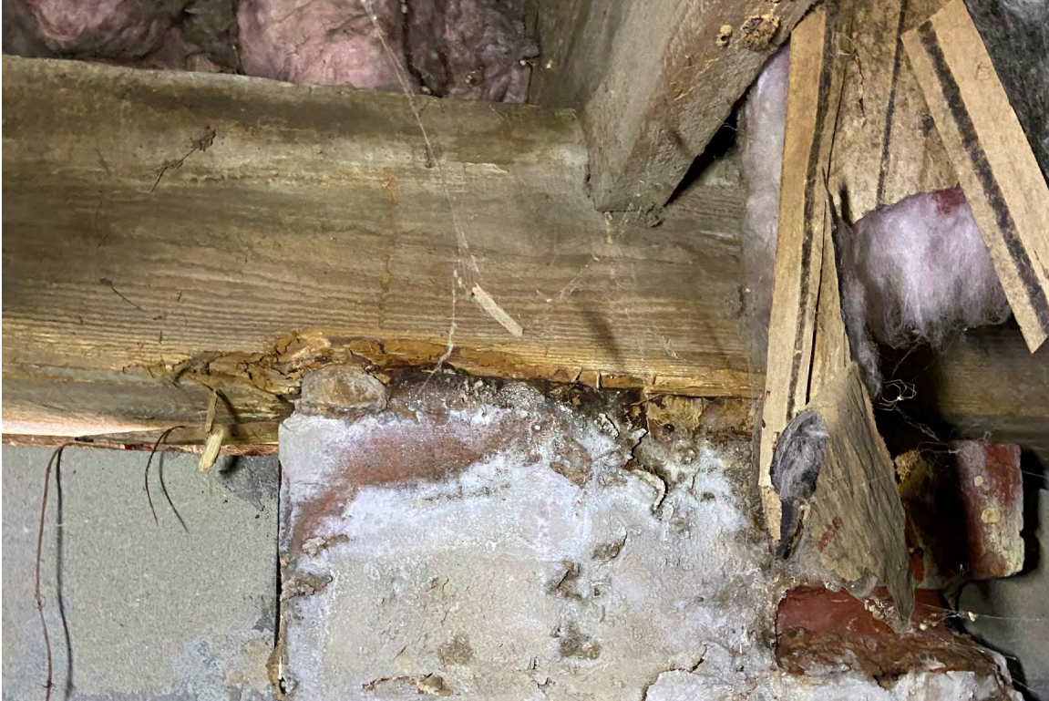
Figure 11: Epps-McGill Farmhouse - PHASE 01: Select girders are crushed and require repair (Kalen McNabb 2020).
