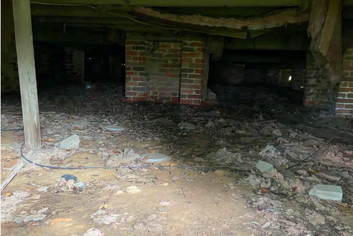
Figure 1: Epps-McGill Farmhouse - PHASE 01: Overview of the crawlspace (Kalen McNabb 2020).
