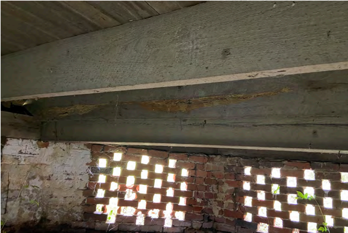
Figure 17: Epps-McGill Farmhouse: Overview of Crawlspace and Joists (Kalen McNabb 2020).
