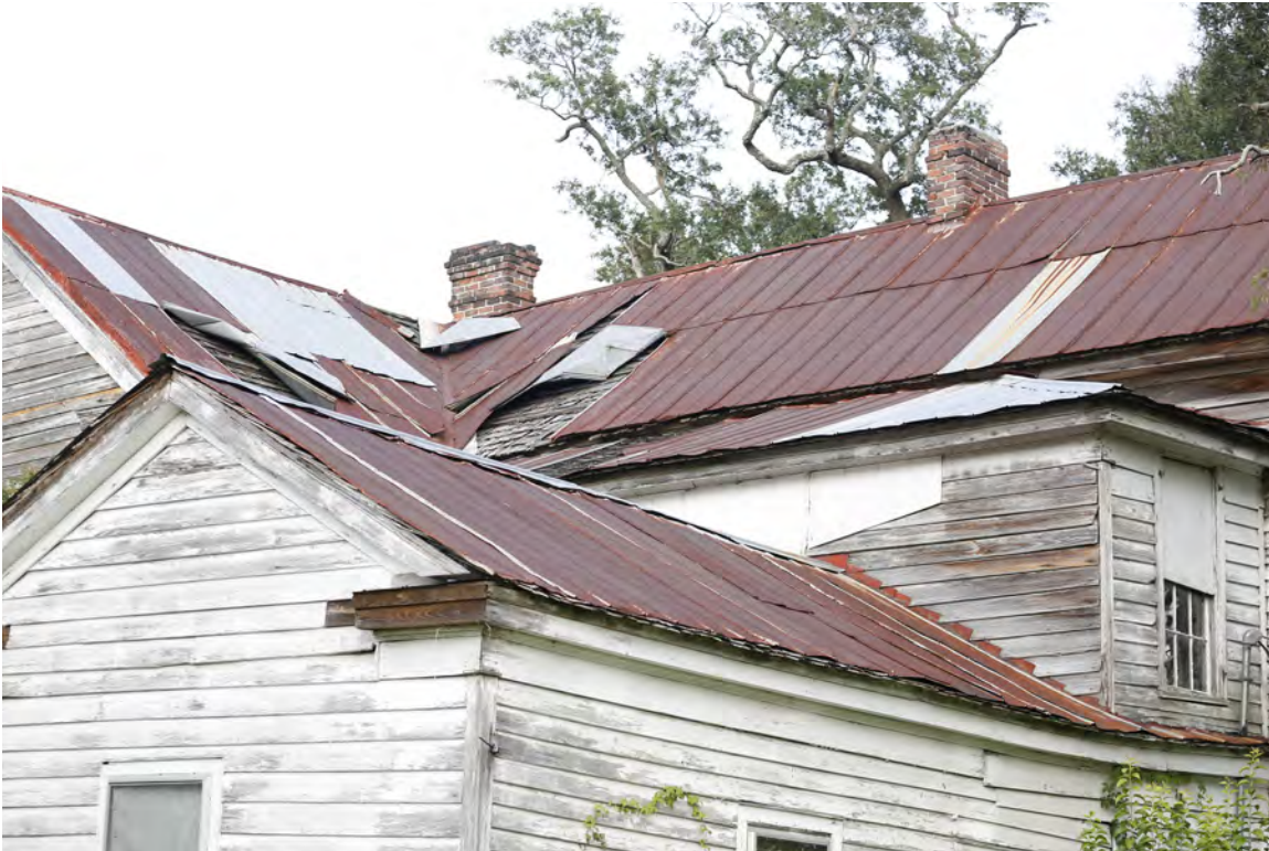
Figure 13: Epps-McGill Farmhouse: Detail of Roof and Chimneys (Kalen McNabb 2020).
