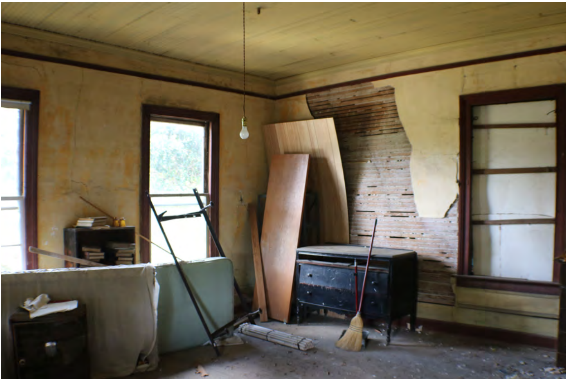
Figure 40: Epps-McGill Farmhouse, Room 206: Second-Floor South Bedroom Looking Southwest (Kalen McNabb 2020).
