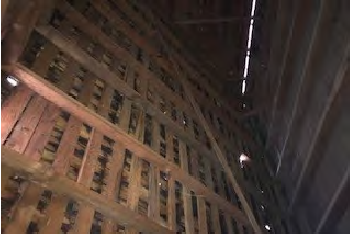
Figure 19: Epps-McGill Farmhouse: Overview of Attic and Framing (Mike Hance 2021).
