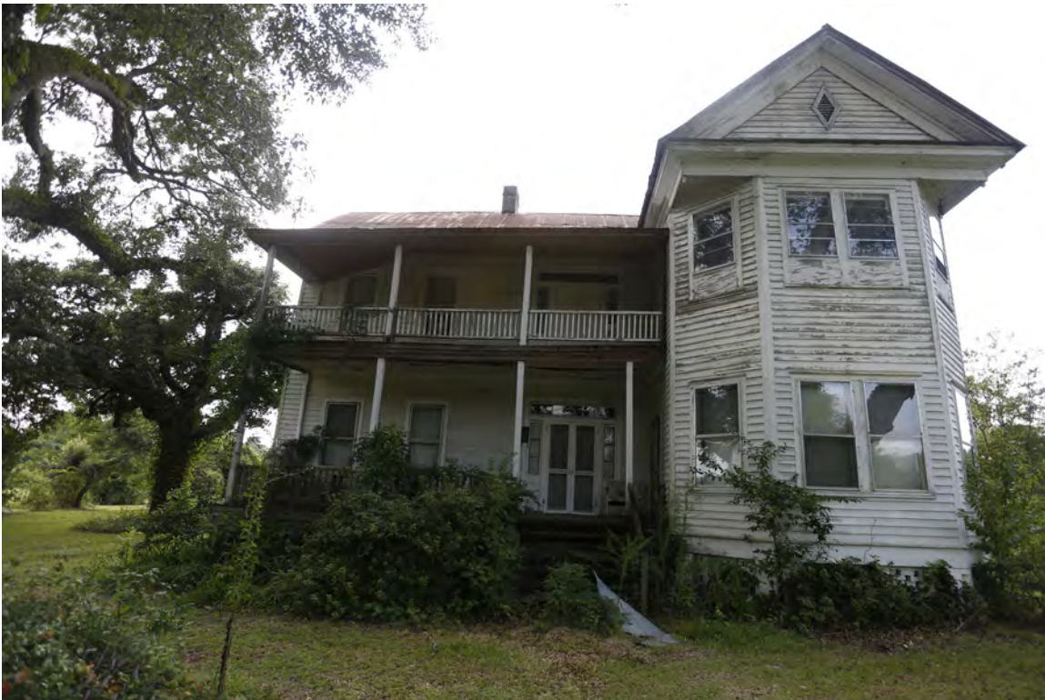
Figure 10: Epps-McGill Farmhouse: East Facade and Porches (Kalen McNabb 2020).
