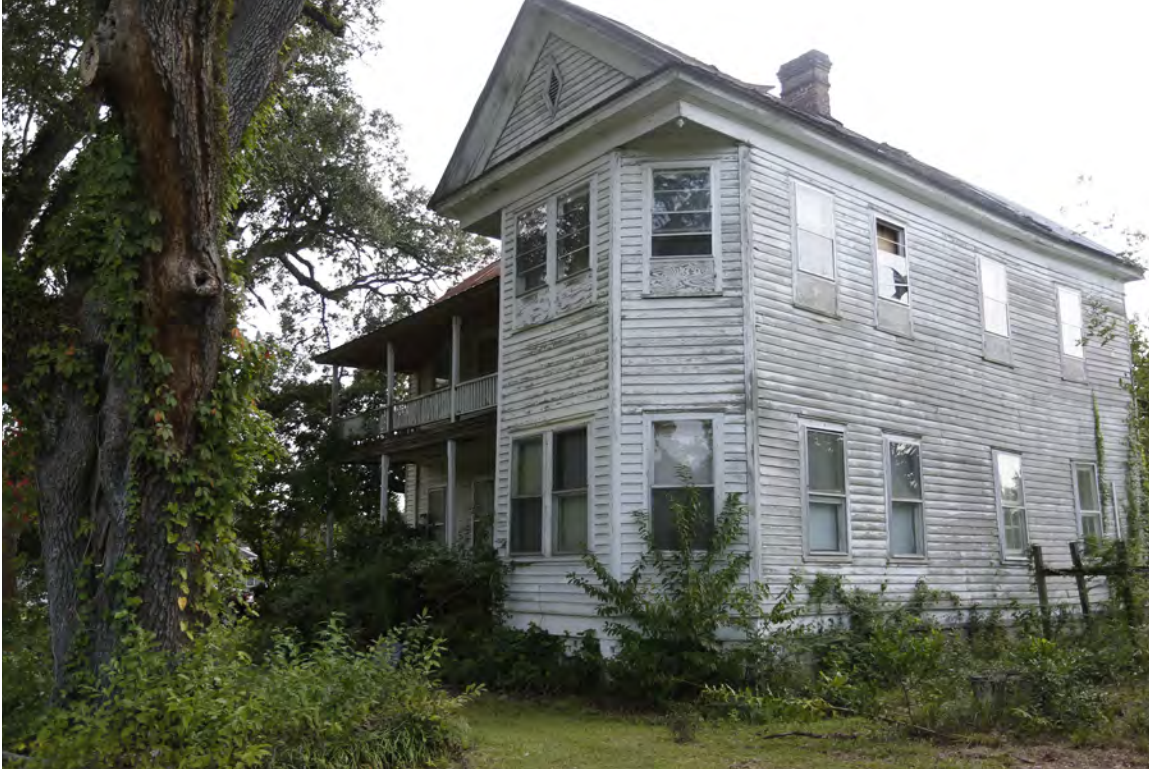
Figure 9: Epps-McGill Farmhouse: Northeast Corner.
