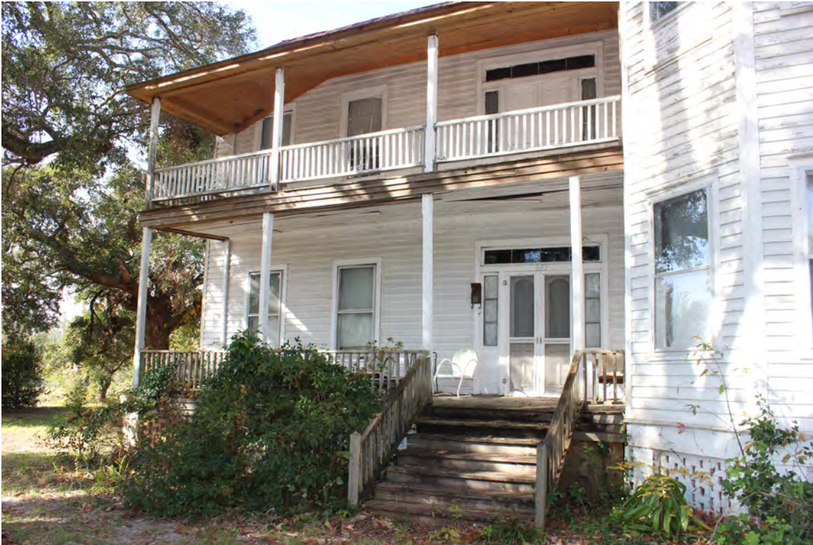
Figure 15: Epps-McGill Farmhouse: Detail of Two-Story East Porch (Kalen McNabb 2020).
