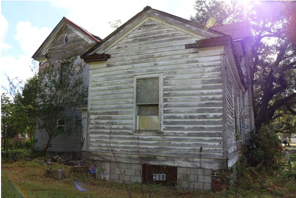
Figure 5: Epps-McGill Farmhouse: West Elevation of Kitchen Building (Kalen McNabb 2020).
