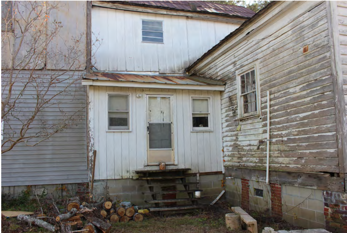
Figure 53: Epps-McGill Farmhouse - PHASE 02: View of location for future deck and ADA access ramp (Kalen McNabb 2020).
