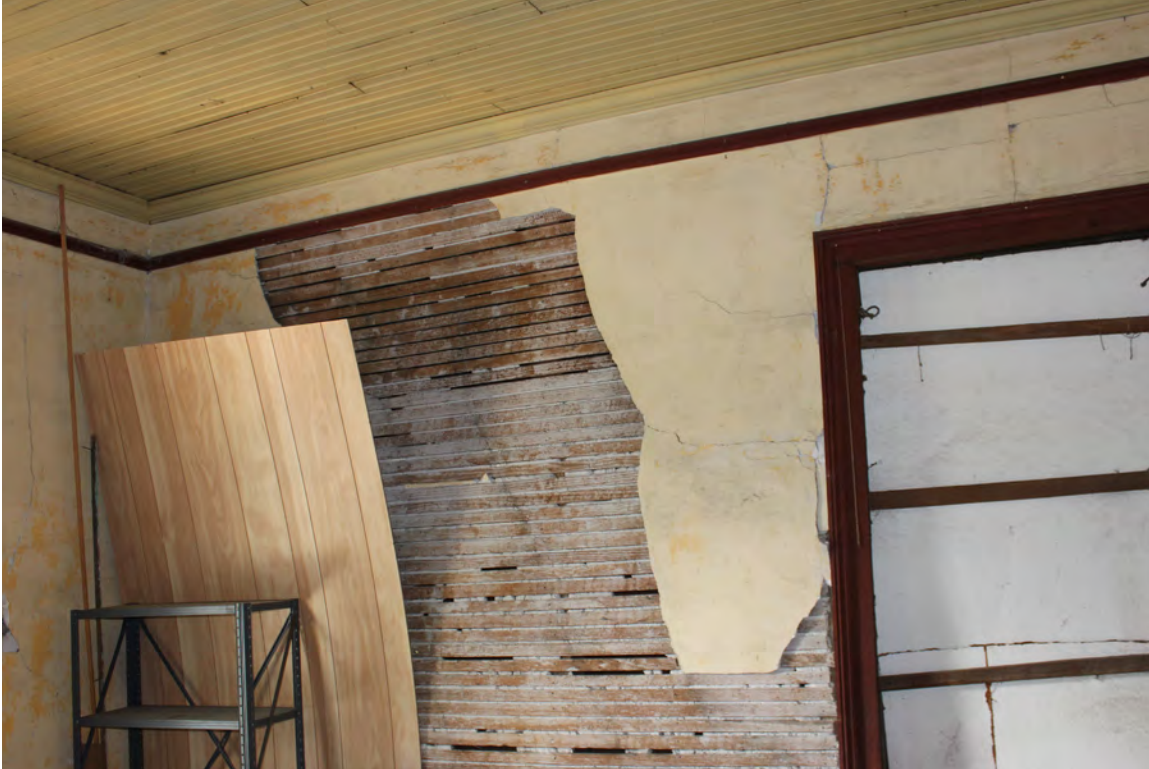
Figure 75: Epps-McGill Farmhouse - PHASE 02: Damaged plaster will be repaired in-kind (Kalen McNabb 2020).
