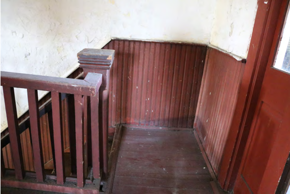
Figure 79: Epps-McGill Farmhouse - PHASE 02: View of second-floor beadboard wainscoting (Kalen McNabb 2020).
