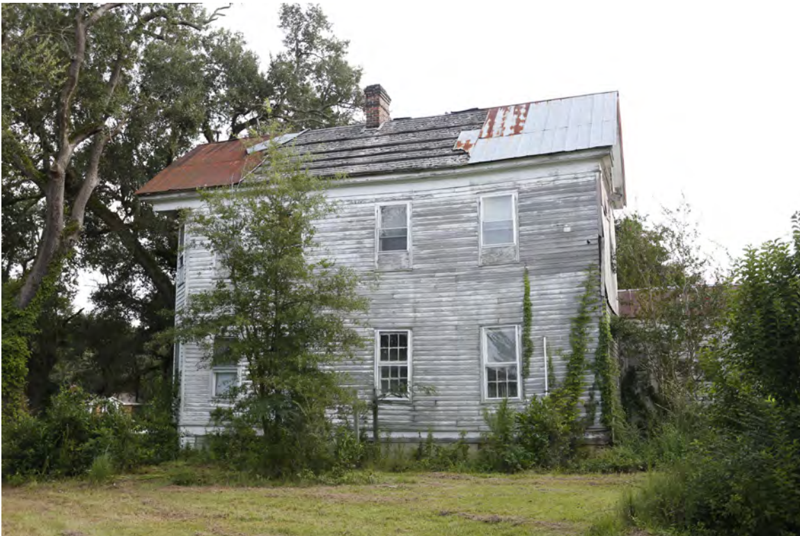
Figure 8: Epps-McGill Farmhouse: North Elevation (Kalen McNabb 2020).
